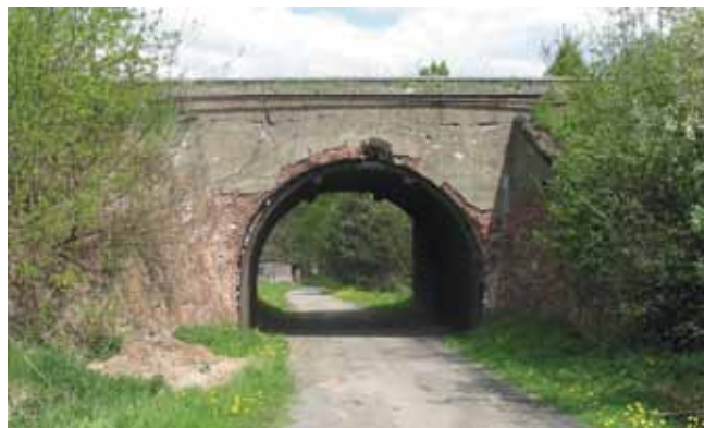
Rys. 1. Ceglany wiadukt łukowy pod torem nr 1 [9] Fig. 1. Brick arch viaduct under railway track no. 1 [9]
