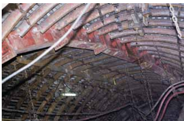
Rys. 21. Obudowa odgałęzienia zabudowana na dole kopalni Fig. 21. Branch support built-up at the bottom of the mine
